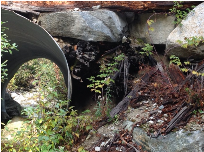
logs as backfill
